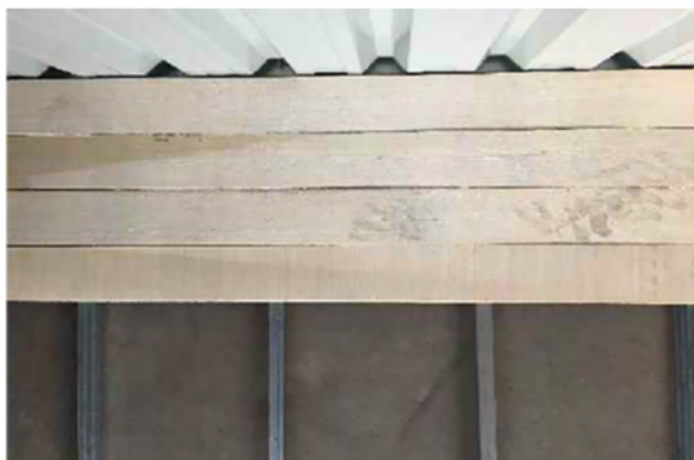
Wood boards added atop floor frame kit.
